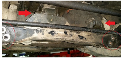
Close up of main X member to be removed & replaced.
