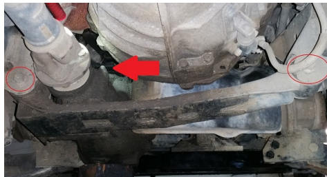
Rear most X member to be removed and fitted with offset bushings
