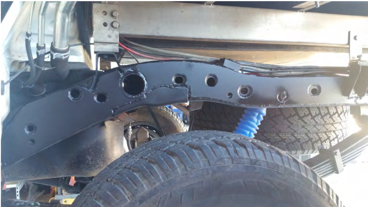
Figure 8: Cleaned, Rust-proofed and painted - Chassis Brace Passenger Side
