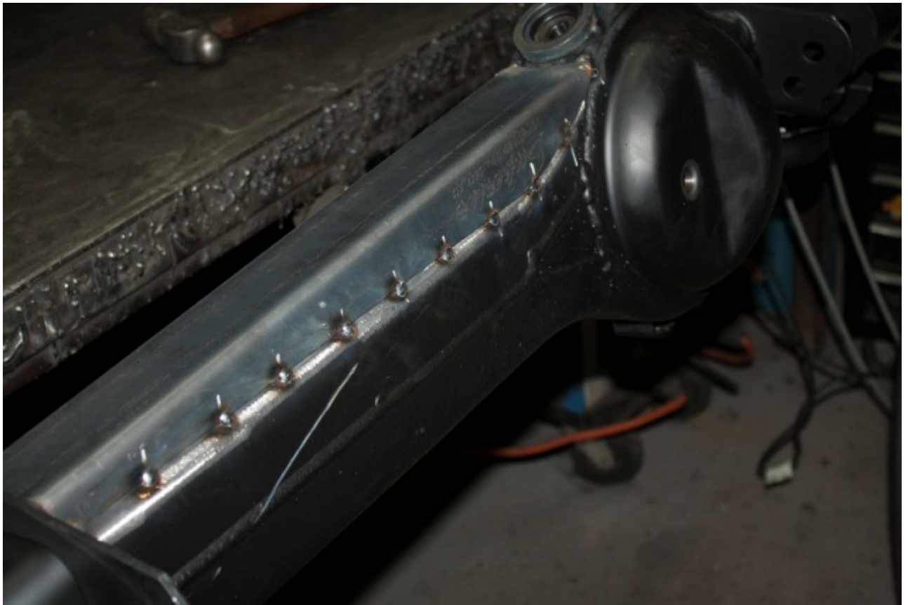
Figure 6: Main Diff Brace Plate Tack Welded In Place
