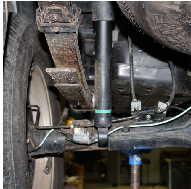
Picture 2: Installation of Raising Block
